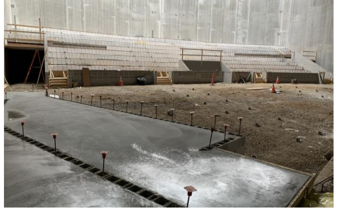
Auditorium floor concrete 10/19/2022
