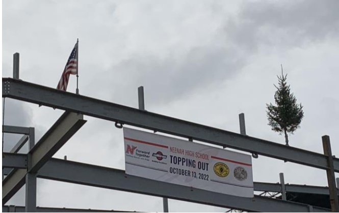
Topping Out – Last piece of structural steel placed 10/13/2022
