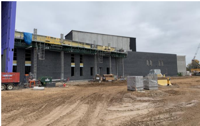
Exterior brick façade on Southeast corner of building 10/19/2022
