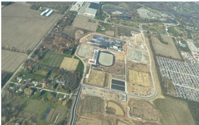
Aerial view of entire project 10/30/2022
